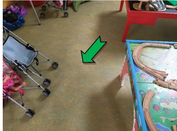
Photo 2. Interior, throughout, floor – non asbestos-containing sheet vinyl.
