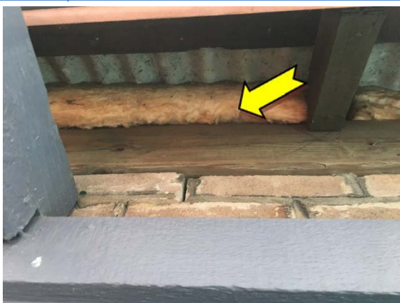
Photo 5. Exterior, between eaves and wall, insulation – suspected SMF sarking insulation material.
